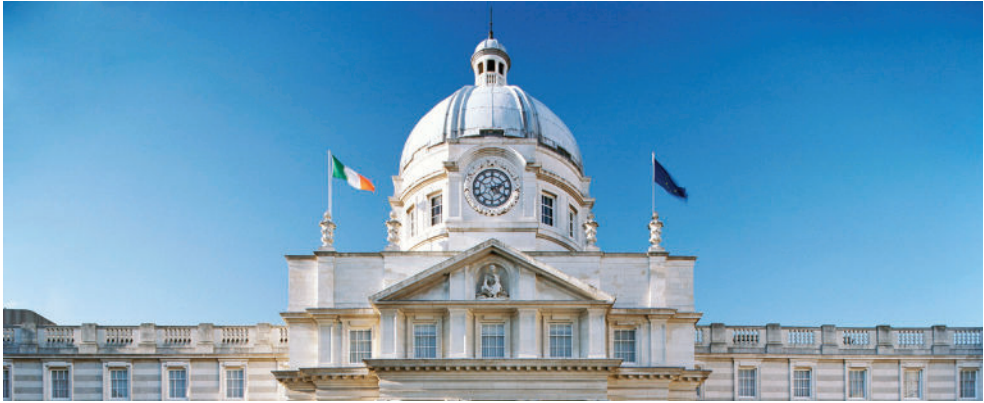
GOVERNMENT BUILDINGS, UPPER MERRION STREET
